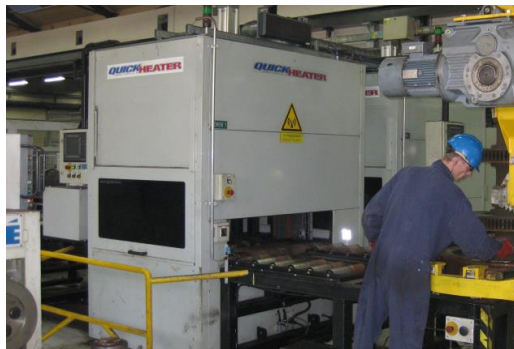
Spot measurements determine control's position
